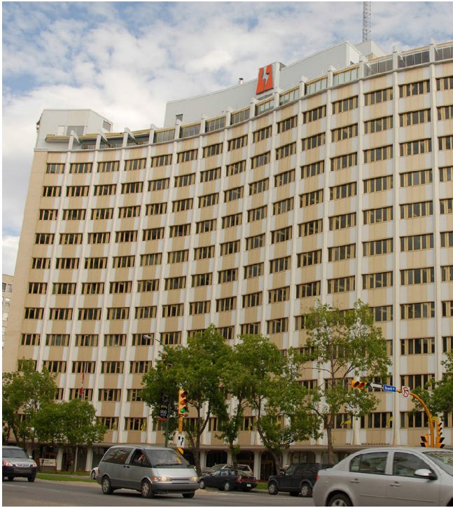
Figure 2: Saskatchewan Power Corporation Head Office Building, c.2000 after being re-clad in aluminum metal panels, SaskPower Archives.
